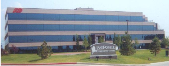
Photo 6-5 New multiple-story commercial structure designed and constructed on helical piles.
