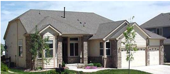
Photo 6-29 Existing residence with settled foundation underpinned and stabilized with helical piles.
