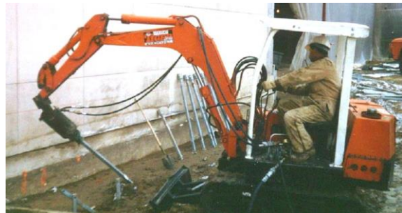
Photo 4-17 Mini-excavator installing battered helical piles adjacent to existing building.
