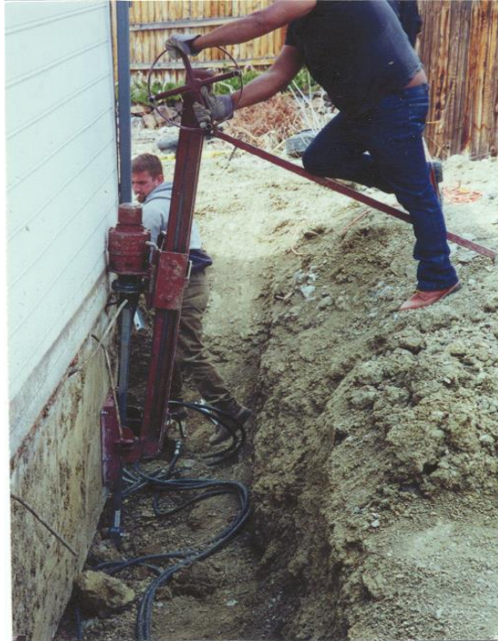
Photo 4-23 Hand-carried mast for installation of helical piles in tight access location.
