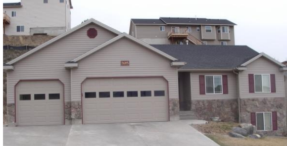
Photo 6-26 Existing residence with settled foundation underpinned/stabilized with helical piles.
