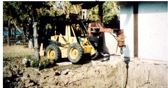
Photo 4-51 Skid-steer mounted torque motor installing helical piles for a new addition.
