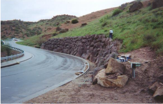
Photo 6-41 New rock faced retaining wall using helical tension anchors as tiebacks.
