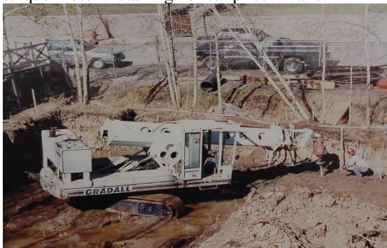
Photo 4-48 Hydraulic excavator mounted torque motor installing helical piles in wet conditions.
