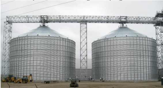
Photo 6-15 New large grain elevator facility designed and constructed on helical piles.
