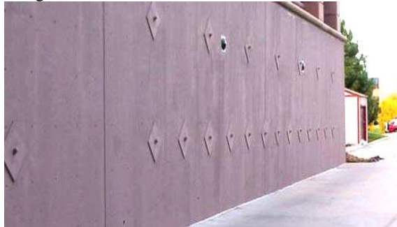
Photo 6-46 Existing foundation/retaining wall laterally supported with helical anchors as tiebacks.
