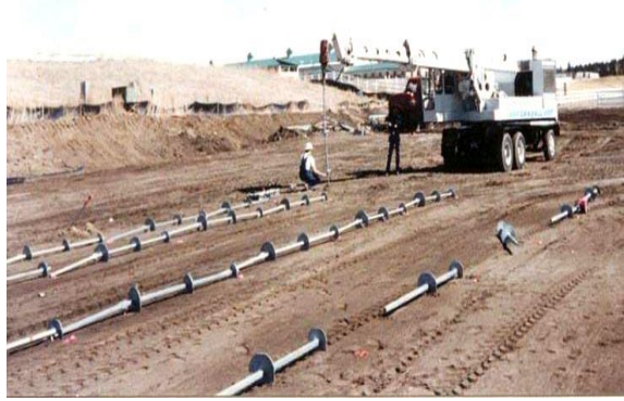
Photo 4-37 Rubber-tire Gradall excavator installing helical piles for new commercial construction.
