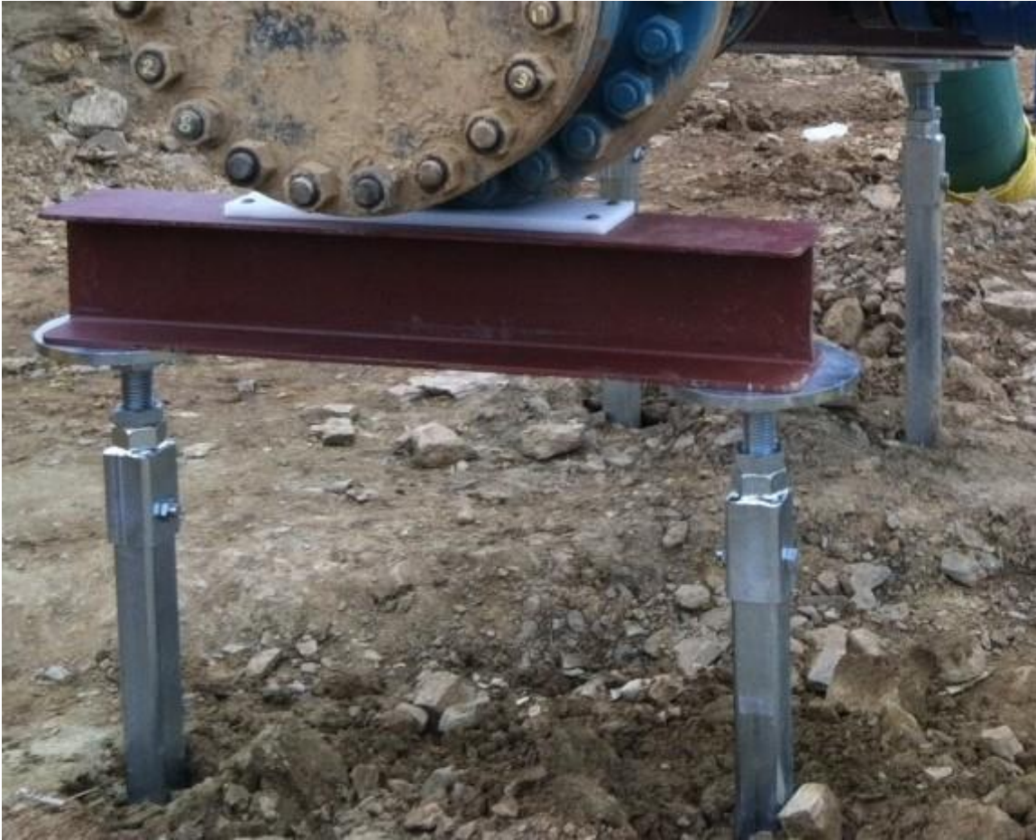
Photo 5-5 Adjustable Equipment/Skid/Pipe Supports on HPFT3 Helical Piles
