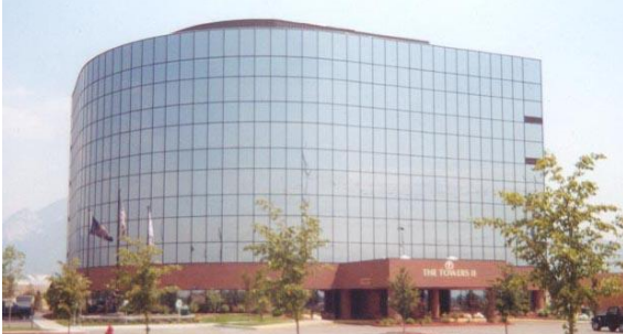
Photo 6-1 New multiple-story commercial structure designed and constructed on helical piles.
