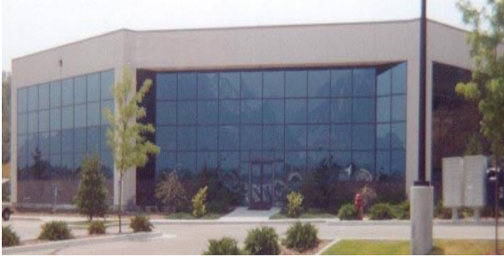
Photo 6-25 Existing building with settled foundation underpinned and stabilized with helical piles.
