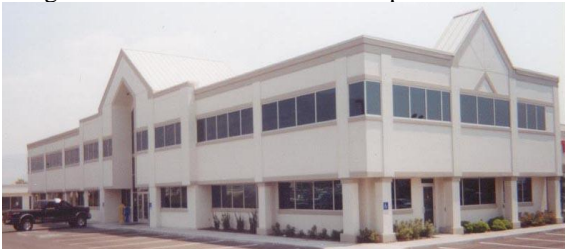
Photo 6-7 New office building designed and constructed on helical piles.
