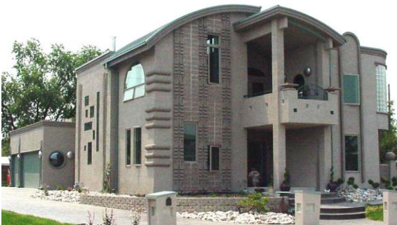
Photo 6-21 New residential structure designed and constructed on helical piles.
