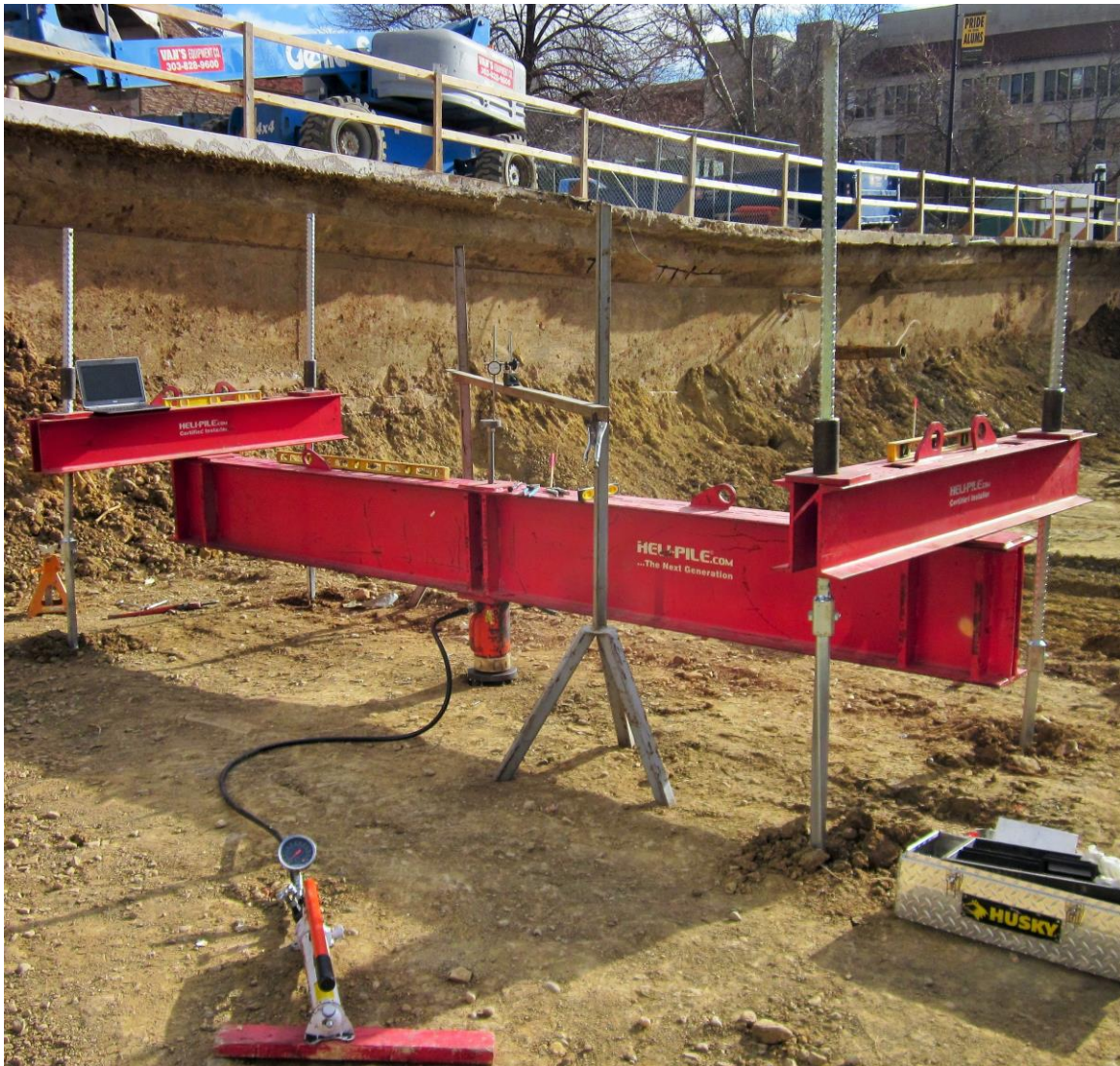
Photo 3-3 Compression load test set-up for a helical pile.
