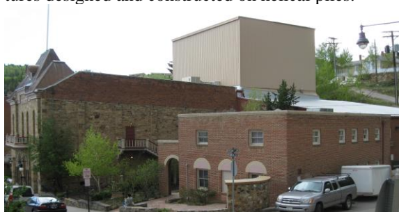
Photo 6-16 New annex to historical structure designed and constructed on helical piles.
