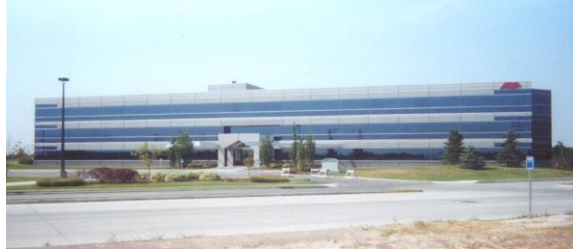
Photo 6-8 New multiple-story commercial structure designed and constructed on helical piles.
