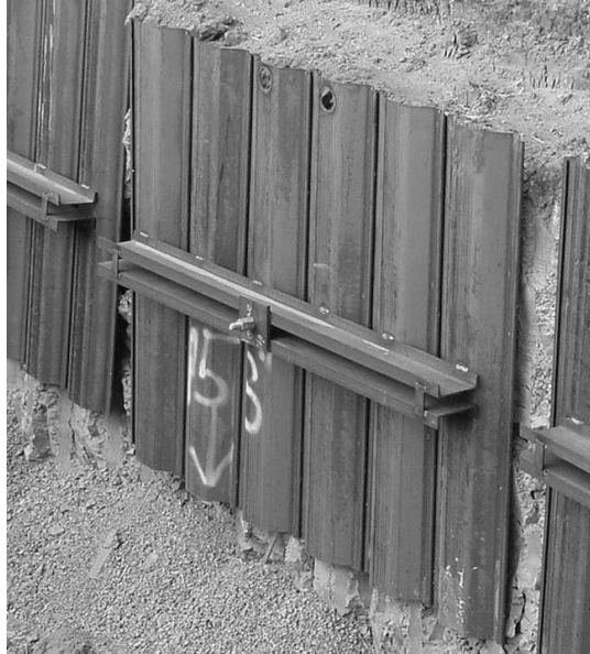
Photo 9-6 Excavation shoring using helical tiebacks and pre-engineered shoring panels.
