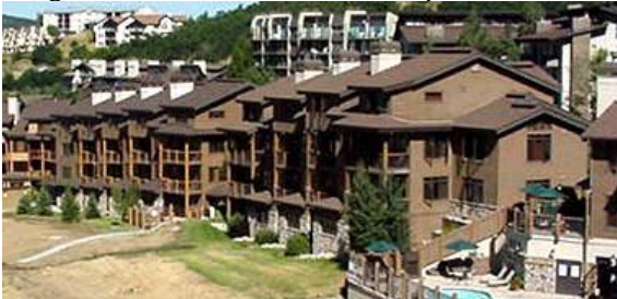
Photo 6-3 New condominium structure in a resort area designed and constructed on helical piles.
