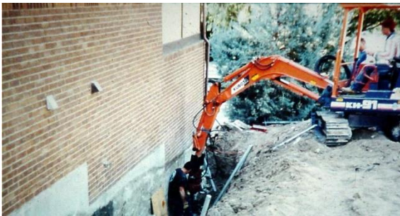
Photo 4-16 Mini-excavator installing helical piles for foundation underpin.
