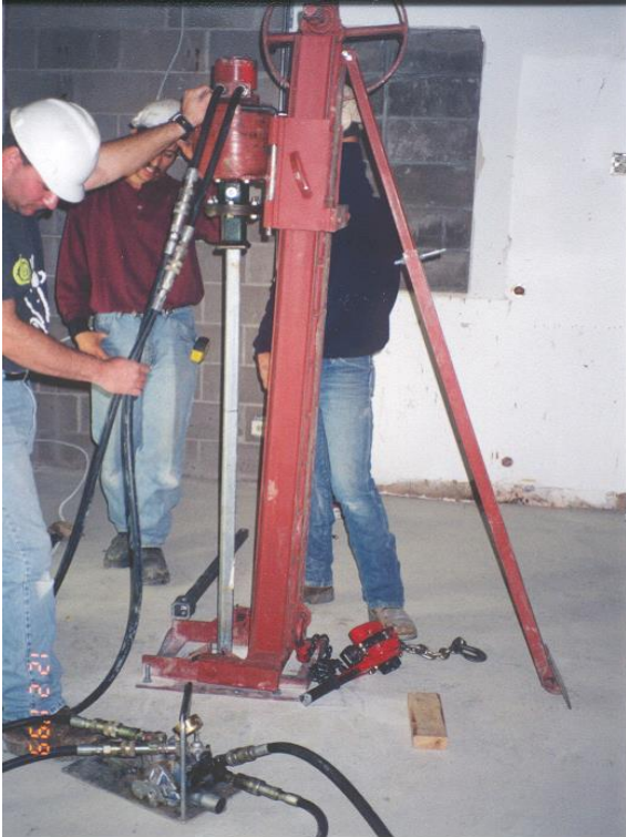
Photo 4-24 Hand-carried mast for installation of helical piles in tight access location.
