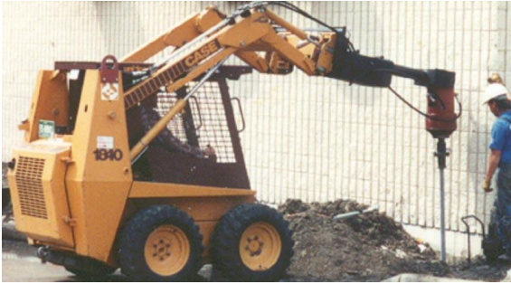
Photo 4-14 Skid-steer machine installing helical piles for foundation underpinning.
