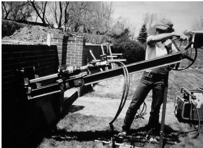
Photo 9-5 Helical tieback in low retaining wall using hand-carried equipment.
