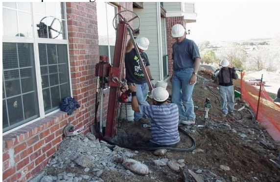
Photo 4-25 Hand-carried mast for installation of helical piles in tight access location.
