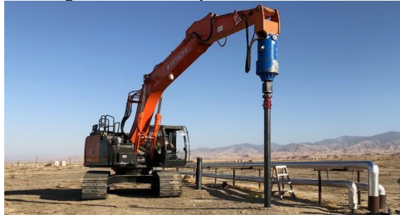
Photo 4-11 Large hydraulic excavator capable of rapidly installing large diameter helical piles.
