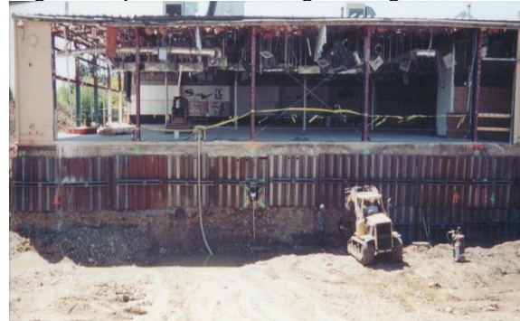
Photo 4-49 Tracked machine installing helical tension anchors as tiebacks for shoring.
