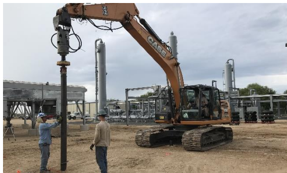
Photo 4-13 Large hydraulic excavator capable of rapidly installing large diameter helical piles.
