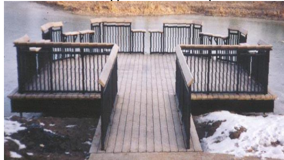
Photo 6-40 New fishing pier supported on helical piles.
