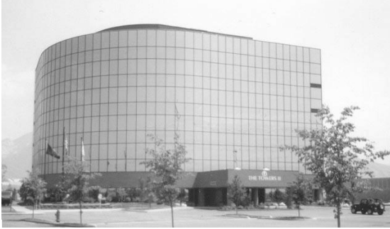
Photo 9-3 Multiple-story bldg on helicals.
