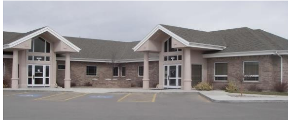
Photo 6-30 Existing building with settled foundation underpinned and stabilized with helical piles.
