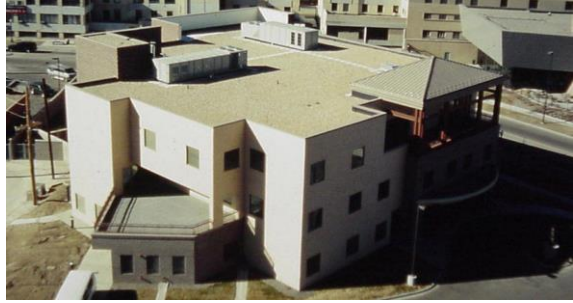
Photo 6-2 New multiple-story commercial structure designed and constructed on helical piles.
