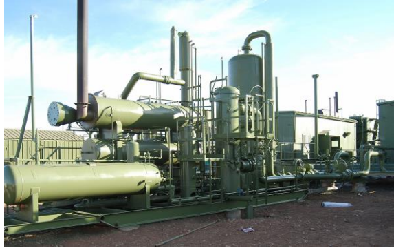
Photo 6-10 New natural gas facility designed and constructed on helical piles.
