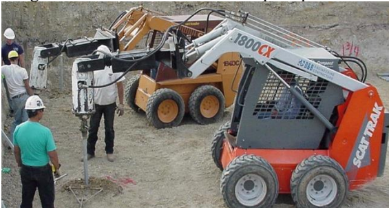
Photo 4-12 Skid-steer type machines installing helical piles for new construction.
