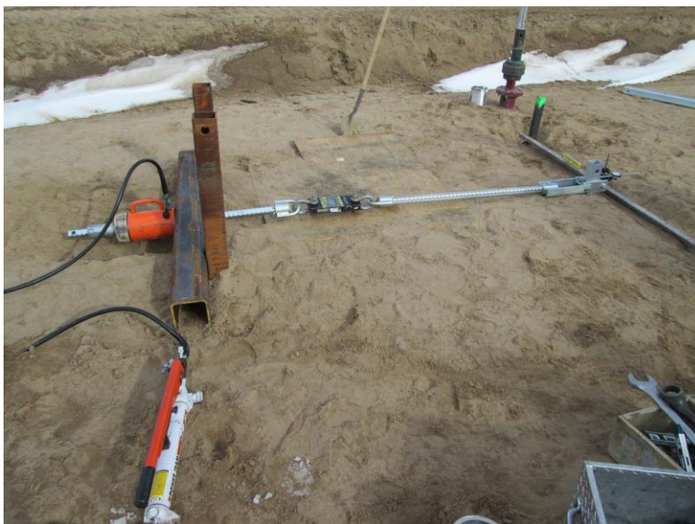
Photo 5-3 Field lateral load test of a helical pile. Test pile at right of photo.
