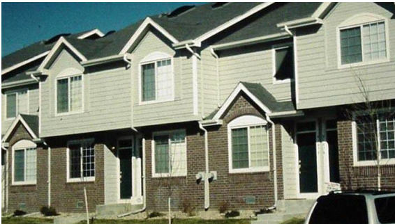
Photo 6-19 New residential condominium structure designed and constructed on helical piles.
