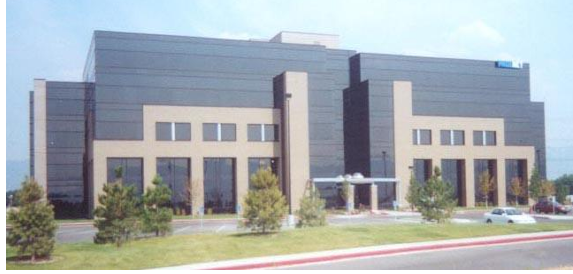
Photo 6-4 New multiple-story commercial structure designed and constructed on helical piles.
