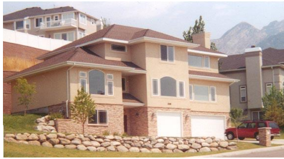
Photo 6-20 New residential structure designed and constructed on helical piles.
