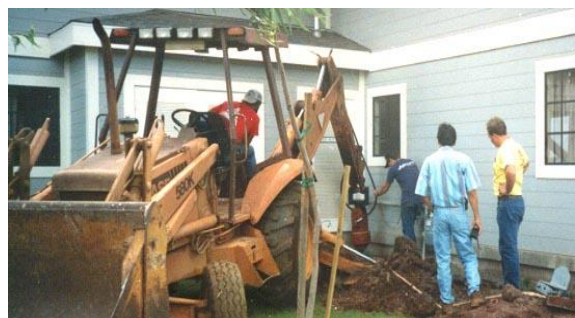
Photo 4-19 Backhoe installing helical piles for foundation underpinning.
