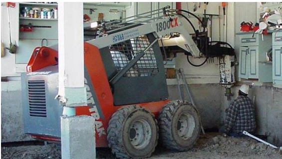
Photo 4-18 Skid-steer machine inside garage installing helical piles for foundation underpinning.
