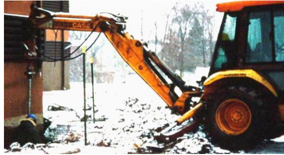
Photo 4-15 Backhoe installing helical piles for foundation underpinning.
