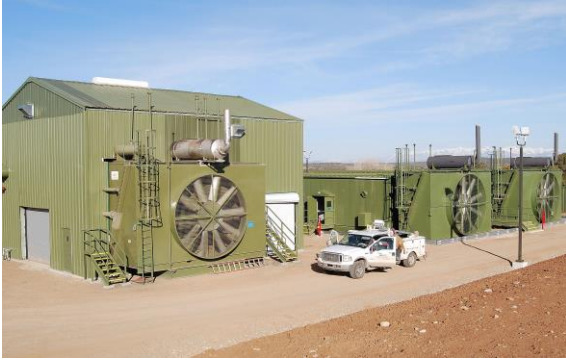
Photo 6-9 New natural gas compressor station designed and constructed on helical piles.
