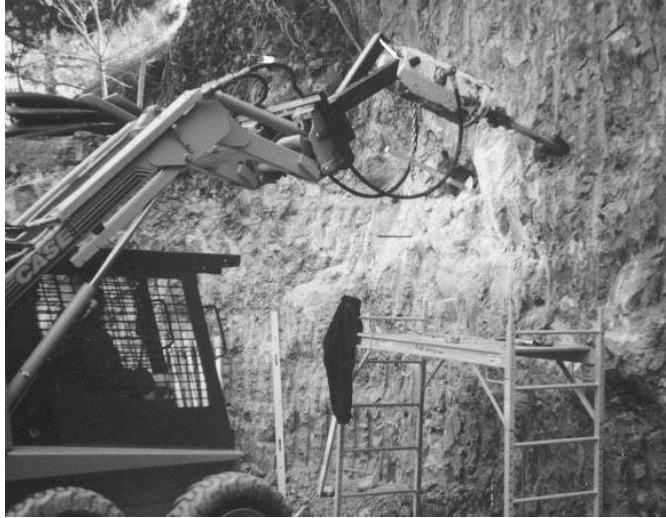
Photo 9-2 Helical tieback installation with drive head mounted on a skid-steer machine.
