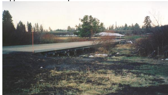
Photo 6-38 New golf cart/pedestrian/vehicle bridge in marsh wetland supported on helical piles.
