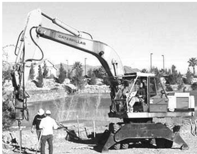
[Paper No. 2] Figure 5. Square Shaft Helical Pier Installation in Expansive Soils. 40,000 lb (178 kN) Machine
