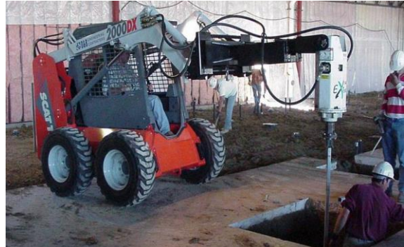
Photo 4-21 Skid-steer machine inside a building installing helical piles for foundation retro-fit
