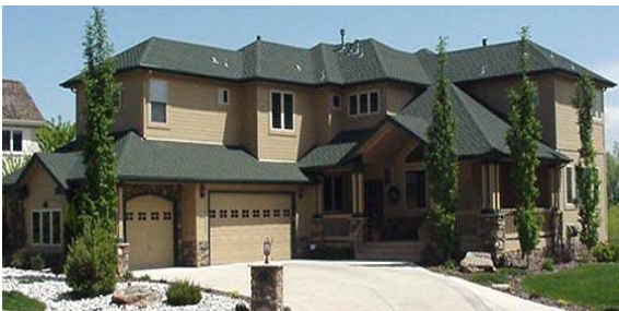
Photo 6-23 New residential structure designed and constructed on helical piles.
