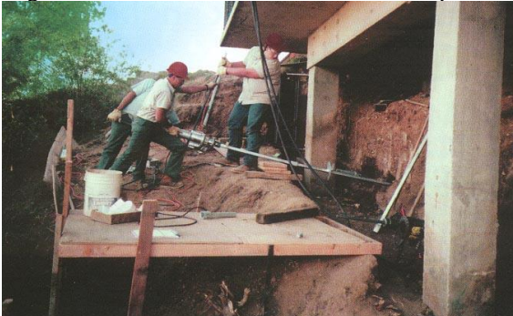
Photo 4-34 Hand-carried equipment installing helical tension anchors as tiebacks for repair.
