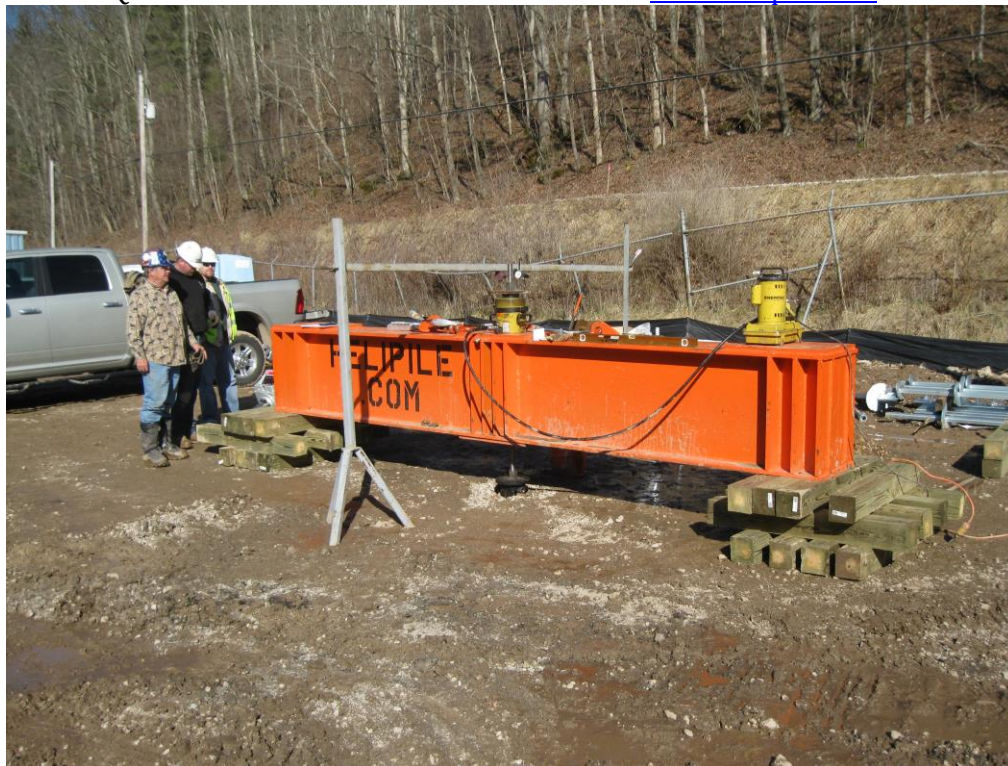
Photo 3-5 Tension load test set-up for Helical Tension Anchor.
