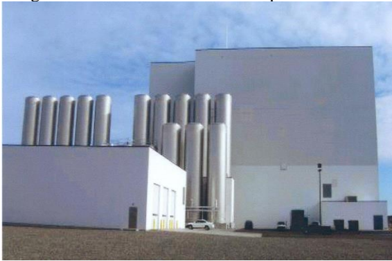
Photo 6-11 New Industrial facility, all structures, including tanks, designed and built on helical piles.
