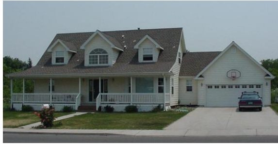
Photo 6-18 New residential structure designed and constructed on helical piles.
