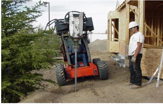
Photo 4-44 Skid-steer mounted torque motor installing helical piles.
