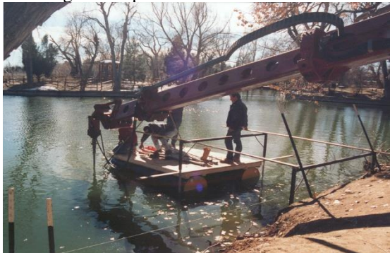
Photo 4-46 Hydraulic excavator boom mounted torque motor installing helical piles in lake.
