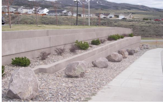
Photo 6-42 New reinforced concrete retaining wall using helical tension anchors as tiebacks.
