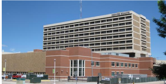
Photo 6-28 The existing nine-story structure was underpinned and shored with helical piles.
