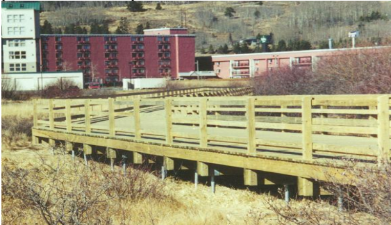
Photo 6-39 New boardwalk in marsh wetland supported on helical piles.
