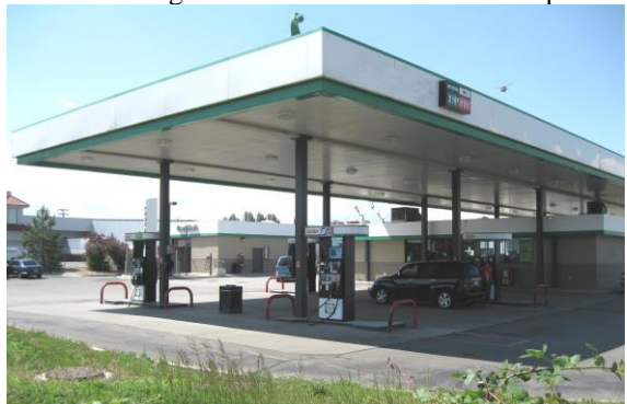
Photo 6-14 New gasoline pump facility. All structures designed and constructed on helical piles.
