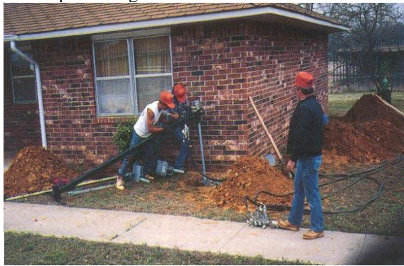
Photo 4-27 Hand-carried torque motor, yoke, and torque arm for tight access location.
