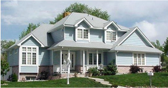
Photo 6-17 New residential structure designed and constructed on helical piles.
