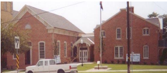
Photo 6-31 Existing rubble foundation under this historic structure replaced using helical piles.
