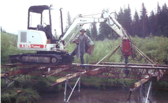
Photo 4-42 Mini-excavator mounted torque motor installing helical screw piles over wetland.
