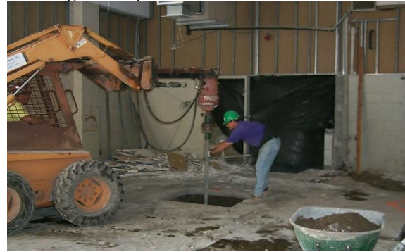
Photo 4-47 Skid-steer mounted torque motor installing helical piles inside existing building.
