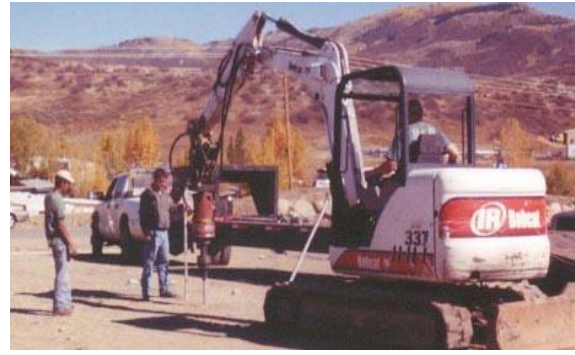
Photo 4-45 Mini-excavator mounted torque motor installing helical piles.
