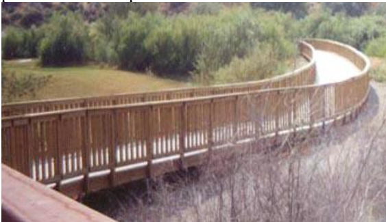
Photo 6-37 New boardwalk in marsh wetland supported on helical piles.
