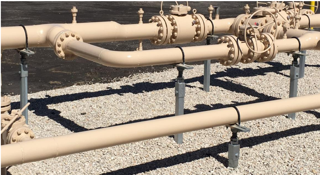
Photo 5-4 Adjustable Pipe Supports on HPFT3 Helical Piles
