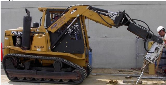
Photo 4-40 Tracked machine installing battered helical piles for lateral load resistance.
