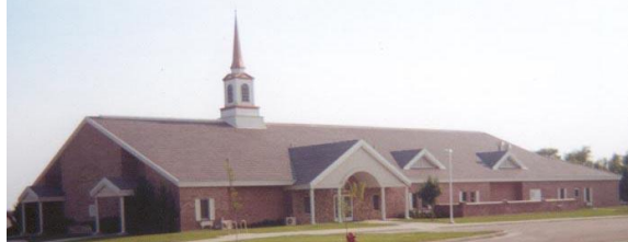
Photo 6-6 New church building designed and constructed on helical piles.
