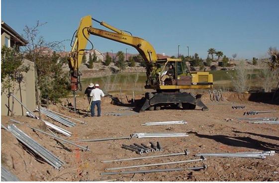
Photo 4-36 Rubber-tire hydraulic excavator installing helical piles for new foundation.
