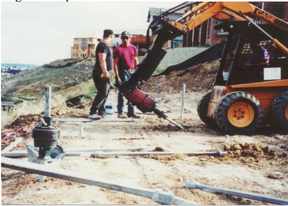
Photo 4-38 Skid-steer mounted torque motor installing battered helical tension anchor under itself.
