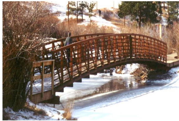
Photo 6-36 New pedestrian bridge with abutments supported on helical piles.
