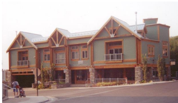
Photo 6-22 New residential condominium structure designed and built on helical piles.
