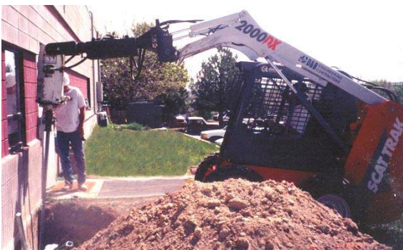
Photo 4-20 Skid-steer machine installing helical piles for foundation underpinning.
