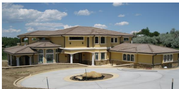
Photo 6-24 New residential structure designed and constructed on helical piles.
