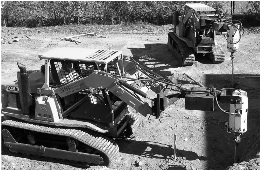
[Paper No. 1] Figure 2. Square Shaft Helical Pier Installation.
