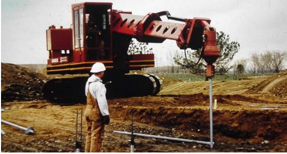
Photo 4-6 Tracked Gradall excavator capable of installing over 60 helical piles per day.
