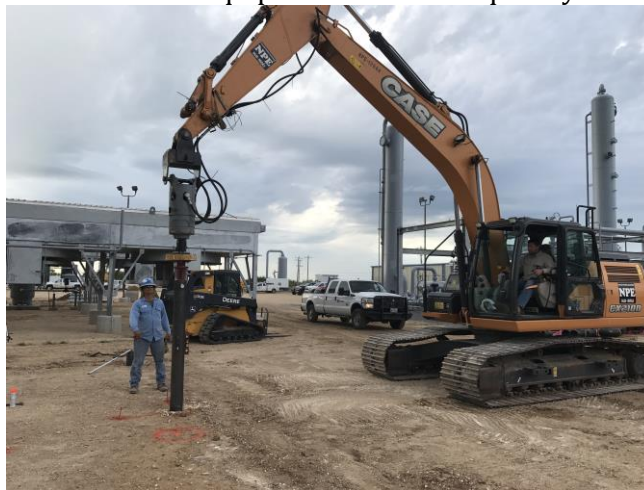
Photo 5-1 Large diameter shaft.
