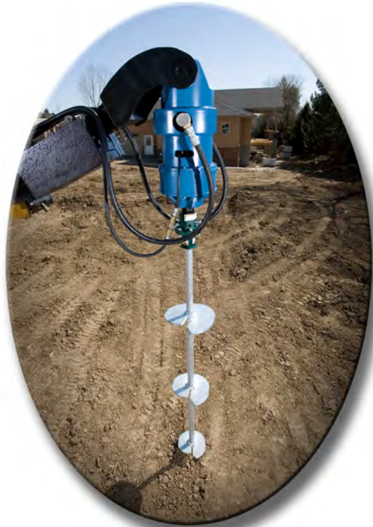
HELI-PILE® Installation
