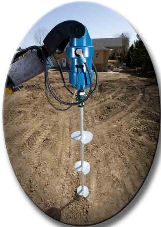
HELI-PILE® Installation
